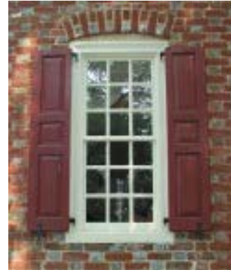
Nine over nine sash window
